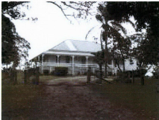
Driveway (Note trees away from house)
